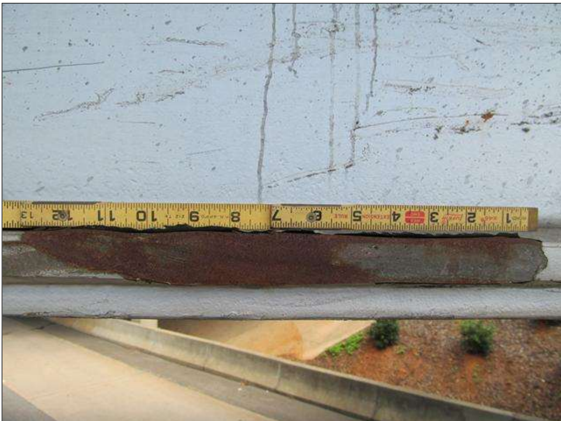
INDENTATION ( 13" X 1/4" ) IN FLANGE ON BEAM 4 @ 21'-2" FROM THE FACE OF BENT 2. BEAM 4, SPAN 3
