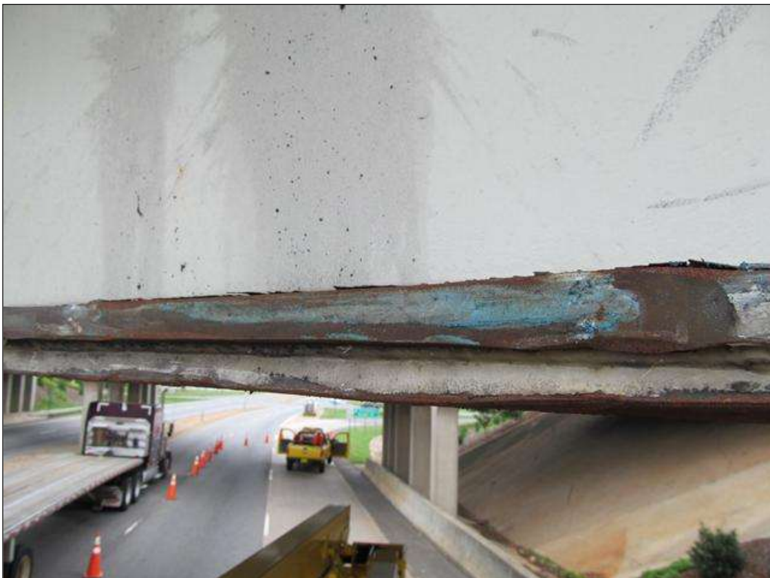
AN INDENTION IN FLANGE FROM 33'-10" TO 24'-4" FROM THE FACE OF BENT 3. BEAM 4,
