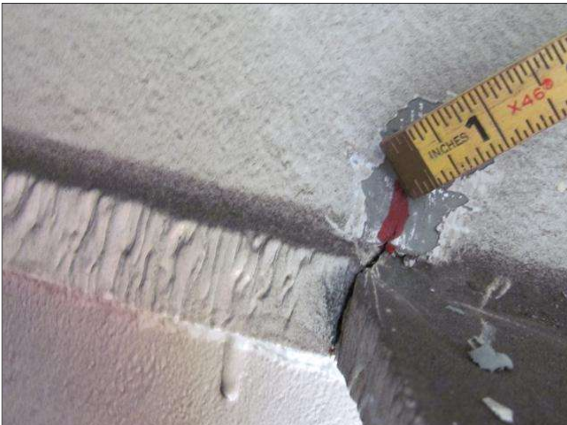
CRACK ( 2" ) IN BOTTOM OF DIAPHRAGM. BEAM 4, SPAN 3
