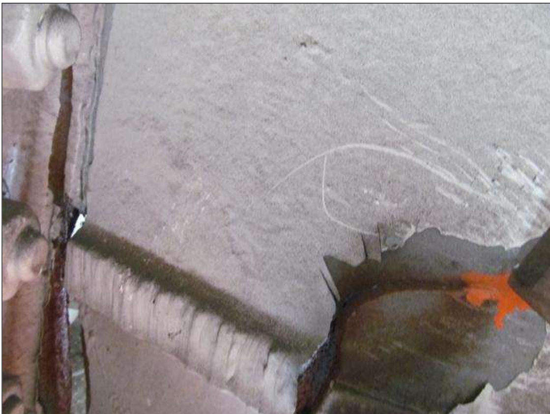
BOTTOM OF DIAPHRAGM @ BEAM 4 HAS A 3 1/2" CRACK. BEAM 4,
