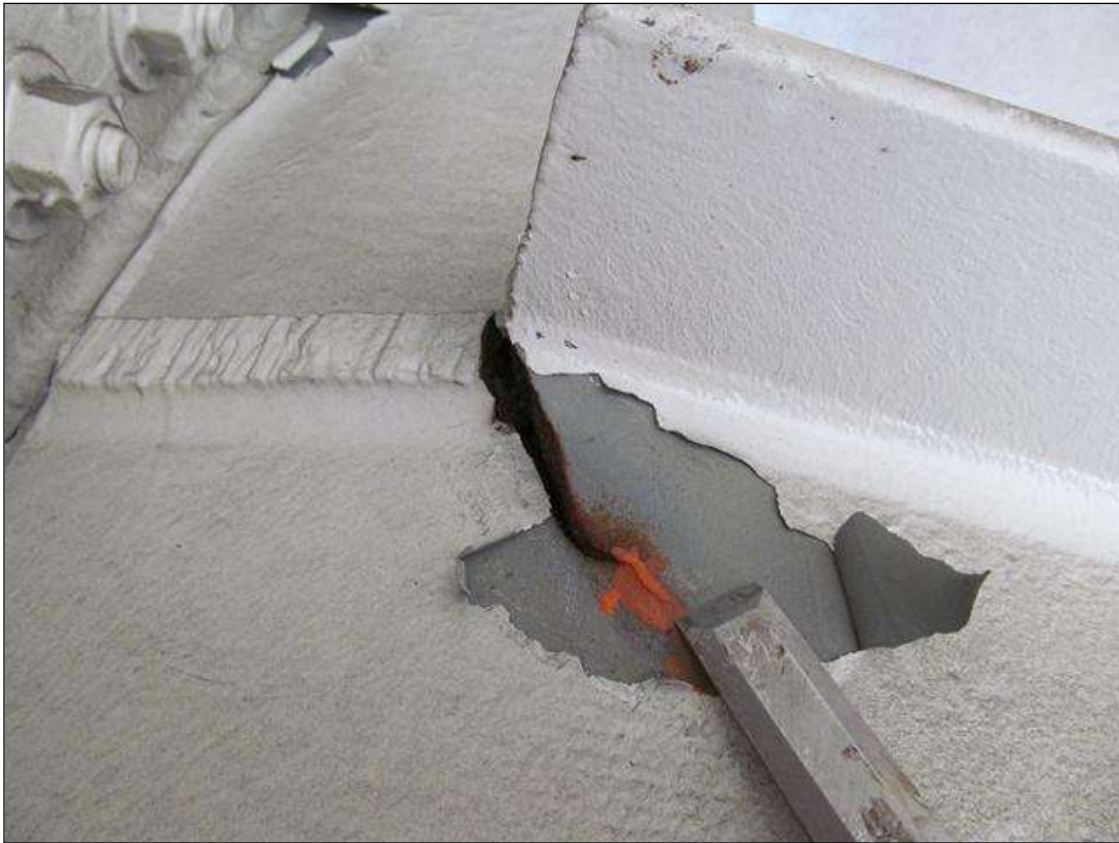
TOP OF DIAPHRAGM @ BEAM 4 HAS A 4" CRACK. BEAM 4,
