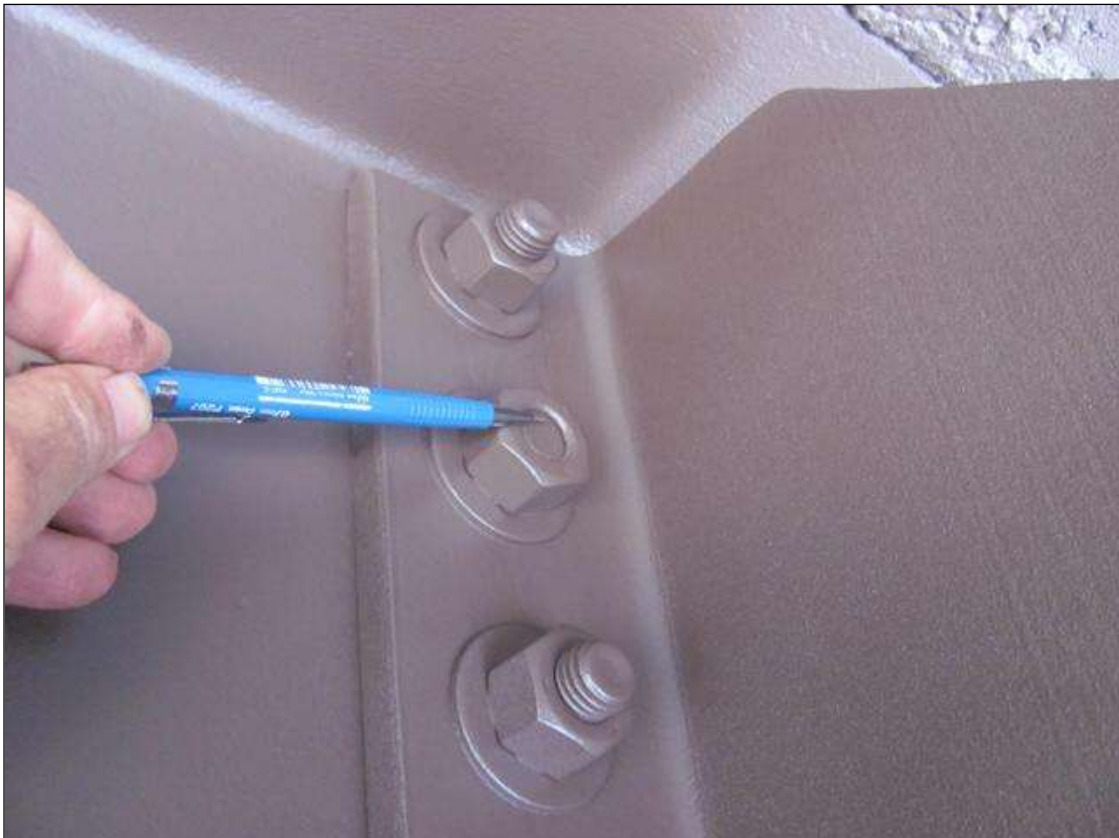
BOLT # 2 ON LEFT SIDE OF DIAPHRAGM @ 16'-6" IS NOT FULLY THREADED. GIRDER 9
