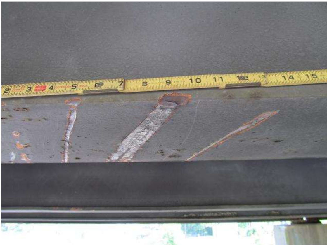
DAMAGE TO BEAM 4 AT 14'-6"
