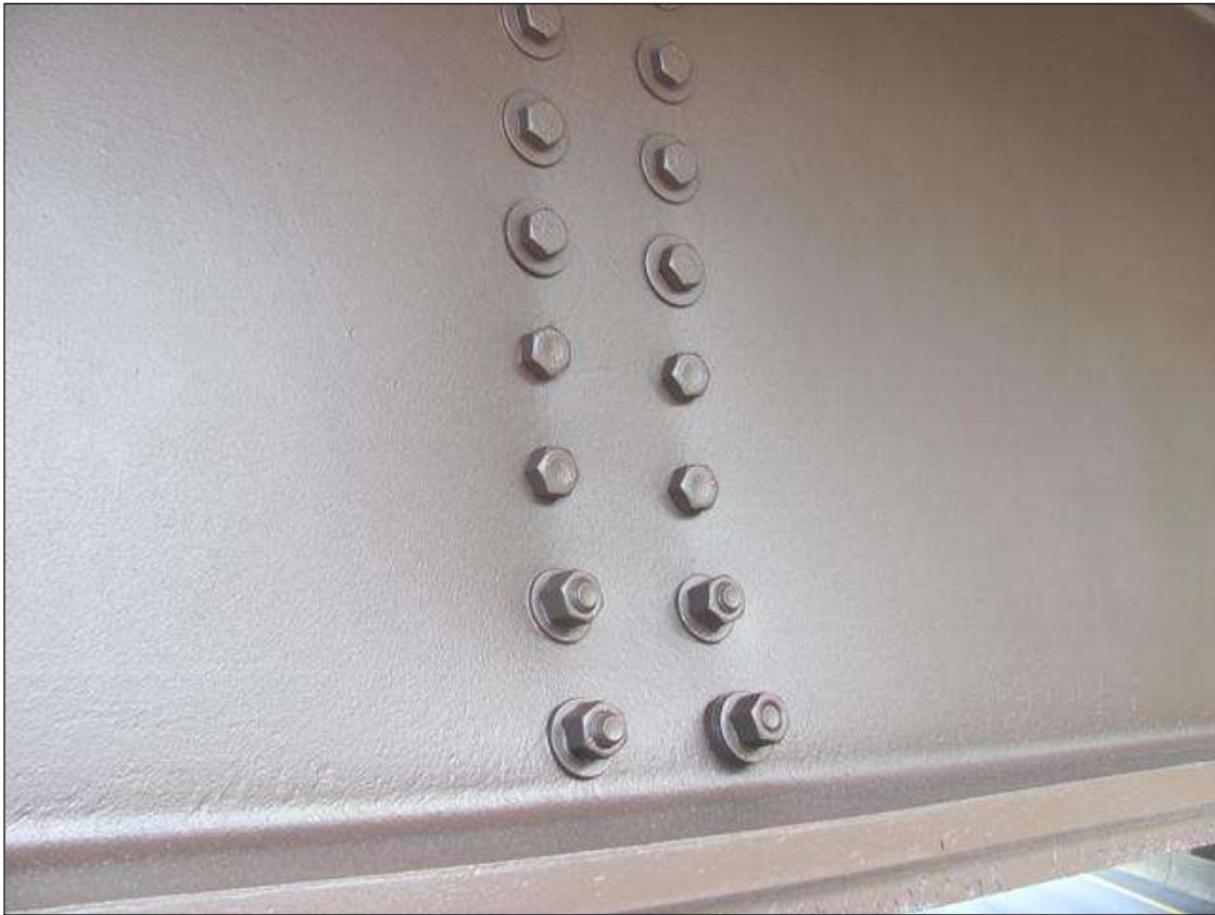
DIAPHRAGM BOLTS ARE LOOSE. FOUR HAVE NO WASHERS. GIRDER 10
