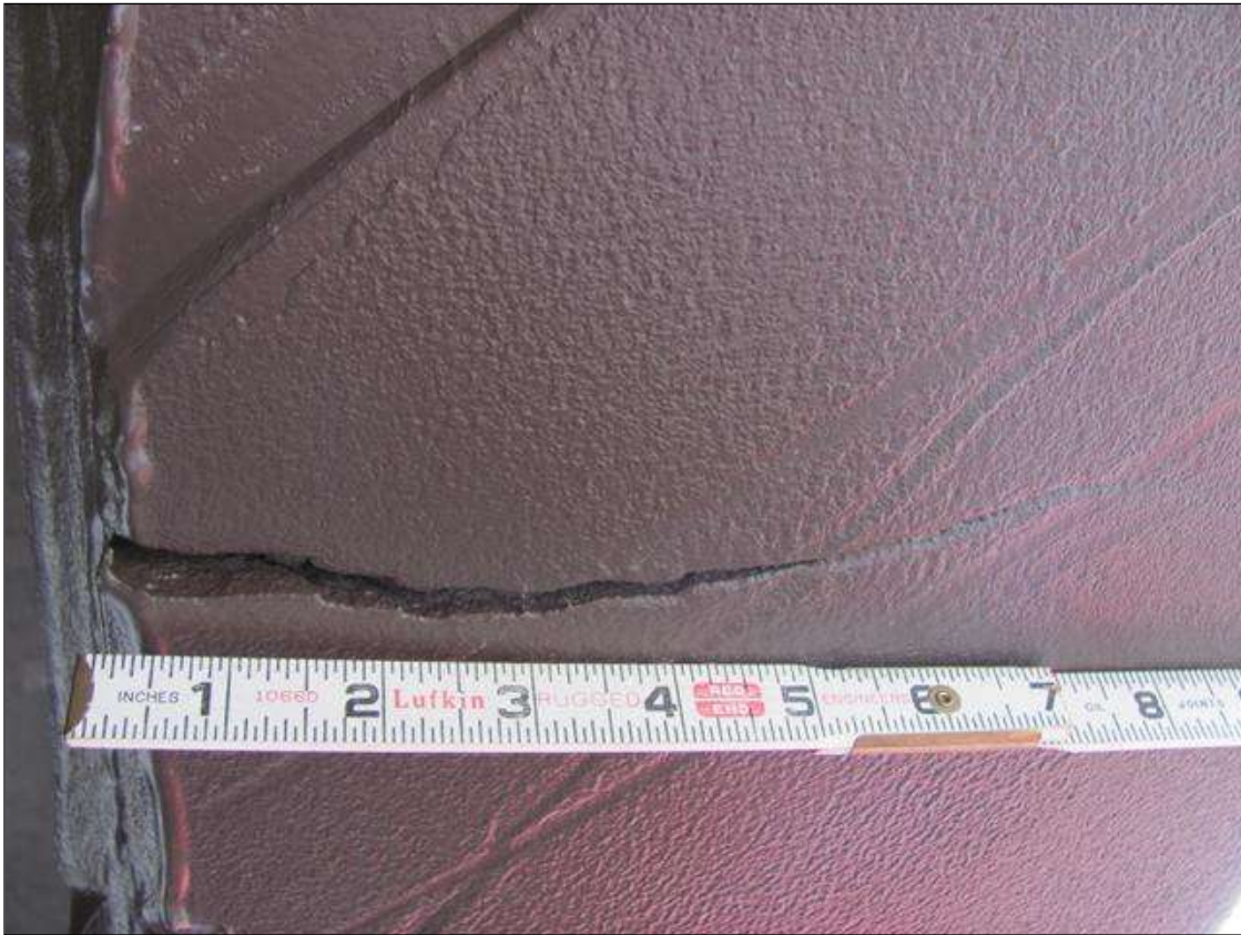
CRACK IN BOTTOM OF COVER PLATE IS 7" LONG. 3 3/4" REMAINS NOT CRACKED. GIRDER 10
