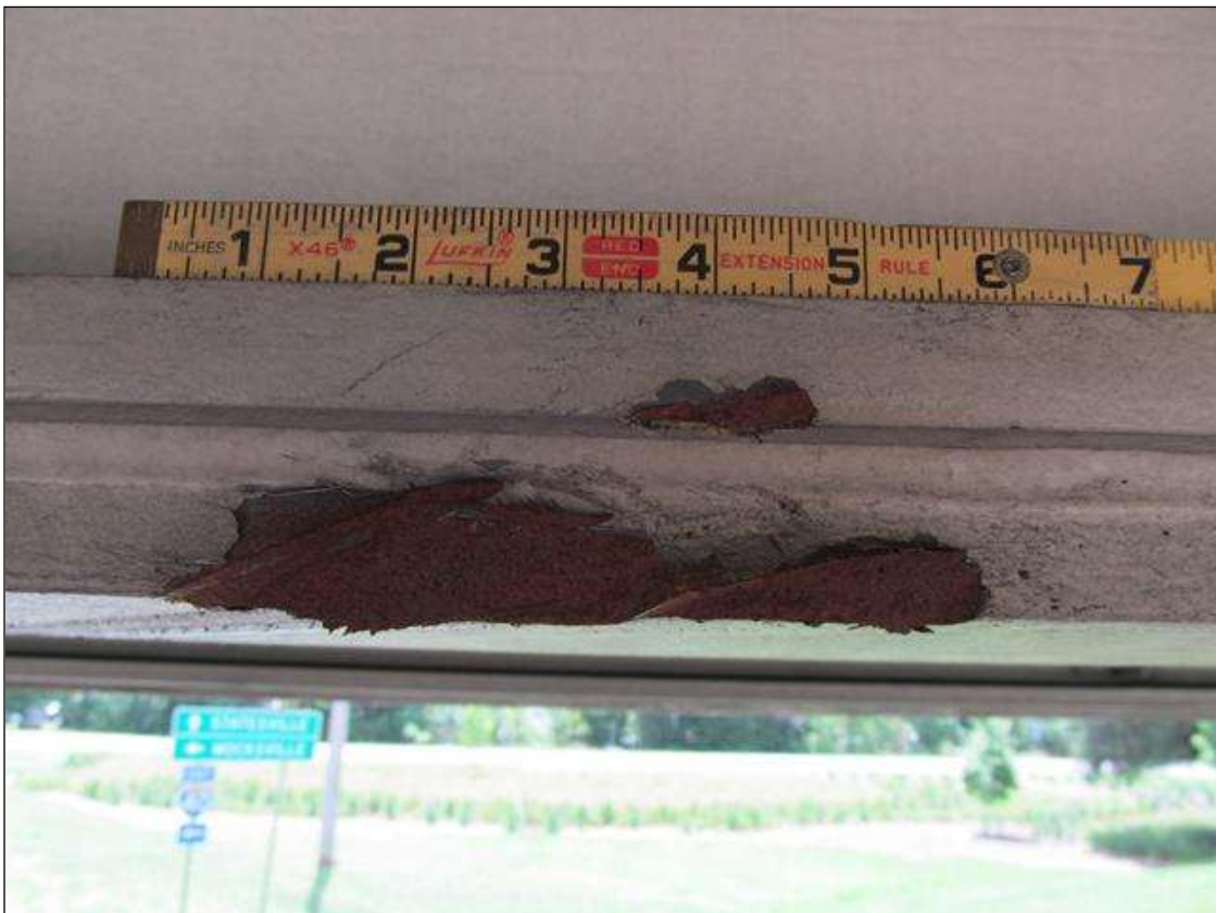
POINT OF IMPACT ON BEAM 2 @ 21'-6" FROM THE FACE OF BENT 2. BEAM 2, SPAN 2
