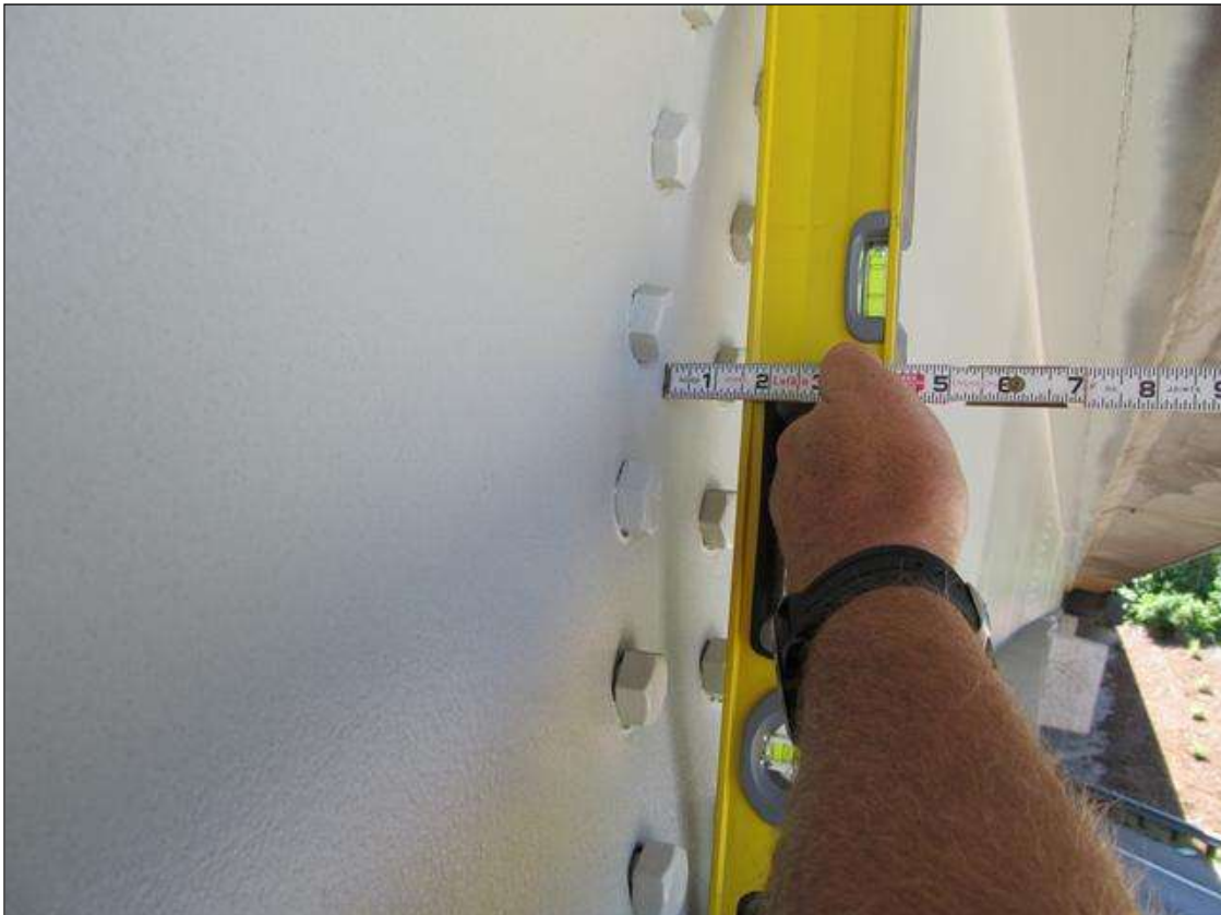
1 1/2" BOW IN GIRDER 10 WEB @ 39'-11" FROM THE FACE OF BENT 1
