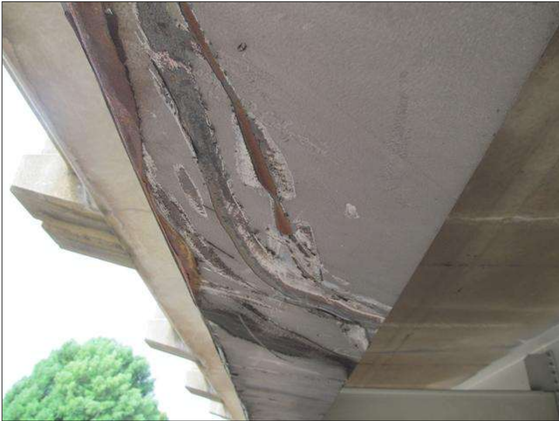
MARKS ON BOTTOM OF COVER PLATE ON BEAM 4 FROM 22'-6" TO 34'-0"
