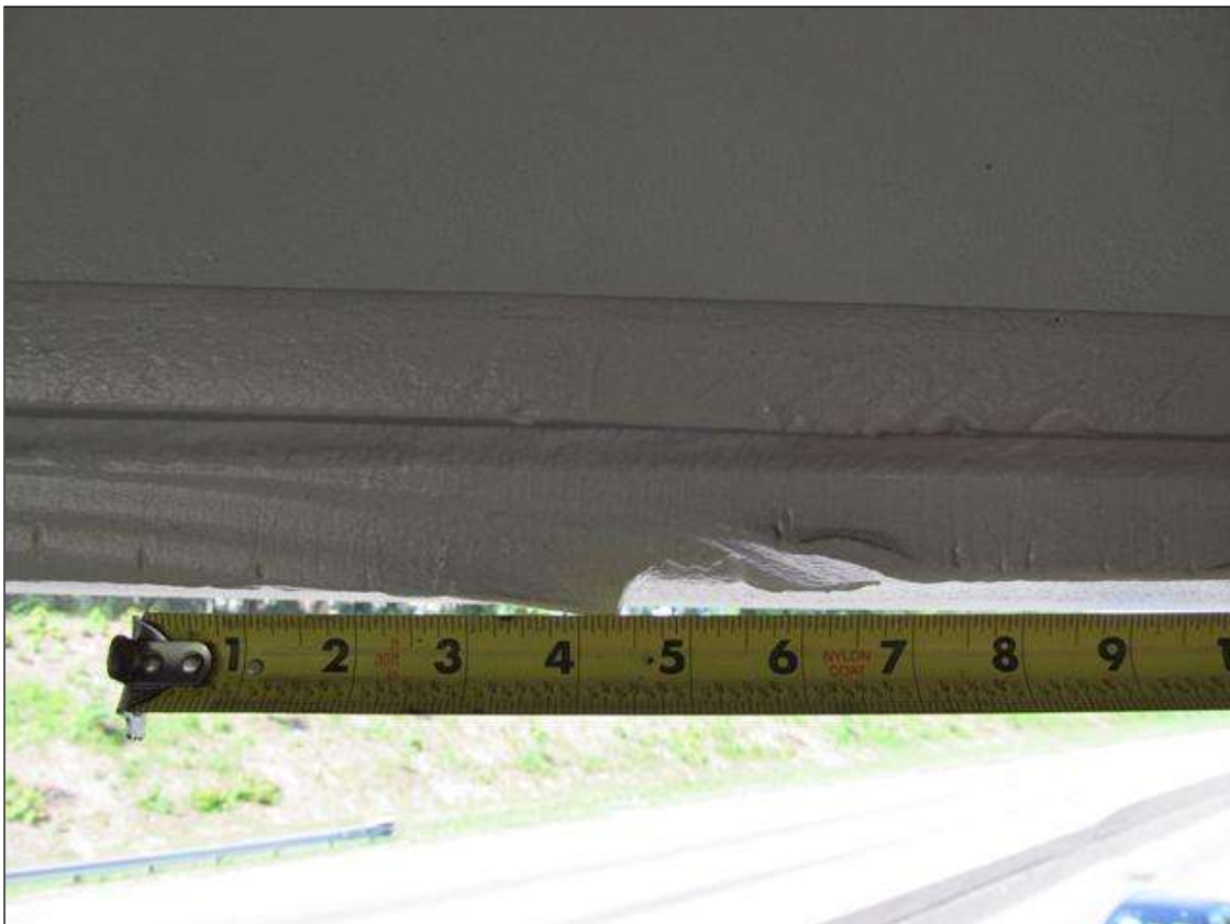
INDENTION ( 7" X 5/8" ) IN COVER PLATE @ 35'-7" FROM THE FACE OF BENT 1. GIRDER 10
