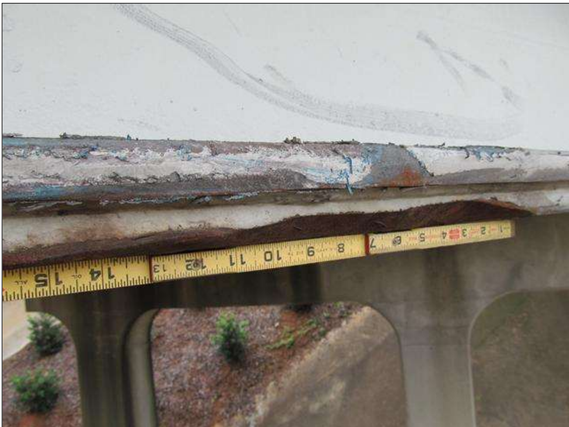
INDENTION ( 48" X 3/4" ) IN COVER PLATE @ 23'-0" FROM THE FACE OF BENT 3. BEAM 4,
