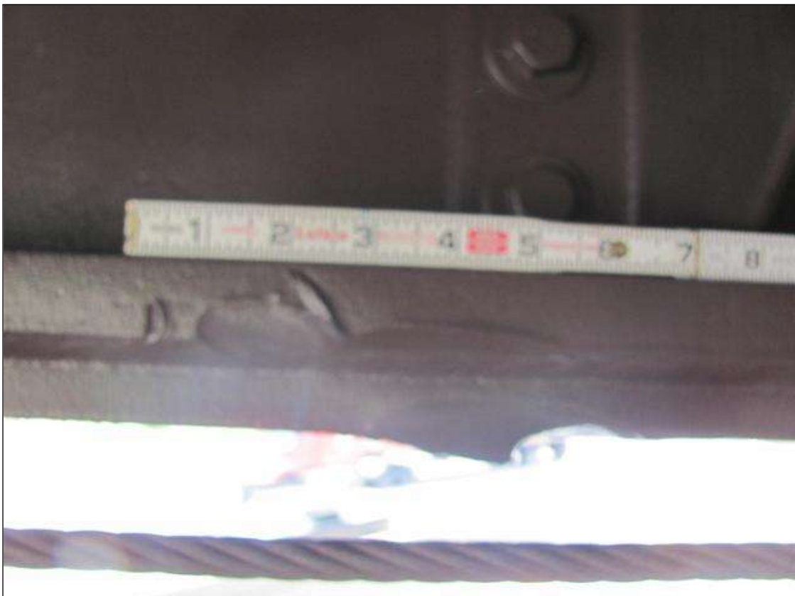
IMPACT ON GIRDER # 7 WAS 23'-11" FROM THE FACE OF BENT 1
