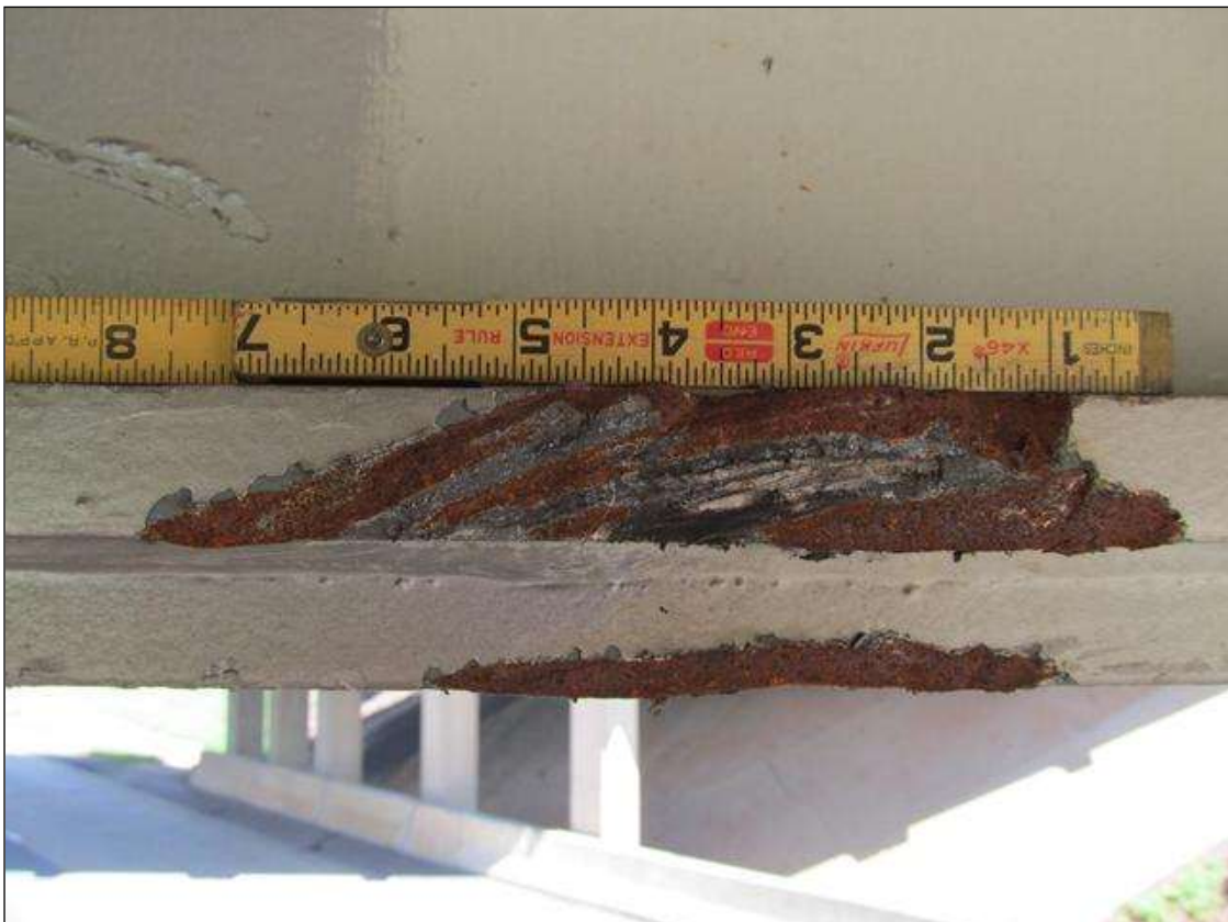
INDENTION IN FLANGE ( 8" X 1/4" ) AND COVER PLATE ( 5" X 1/16" ) @ 14'-5" FROM THE FACE OF BENT 2. BEAM 3, SPAN 3
