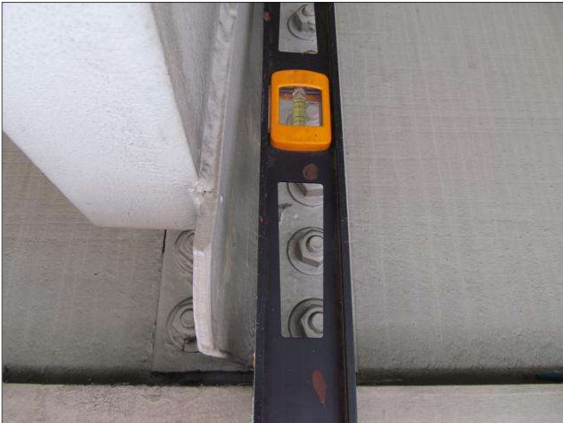
DIAPHRAGM @ 37'-4" FROM THE FACE OF BENT 3, IS OUT OF PLUMB ( 3/4" ) TO THE EAST. BEAM 4, SPAN 3
