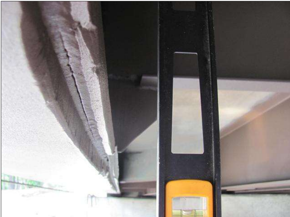
GIRDER 10 IS OUT OF PLUMB 1\frac{7}{8} " IN THE DIRECTION OF TRAFFIC @ 20'-2" FROM THE FACE OF BENT 1.
