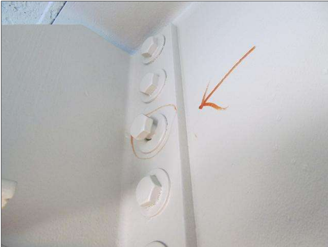
DIAPHRAGM BOLT ON RIGHT SIDE OF GIRDER 9 IS NOT PULLED UP TIGHT @ 34'-7" FROM THE FACE OF BENT 1
