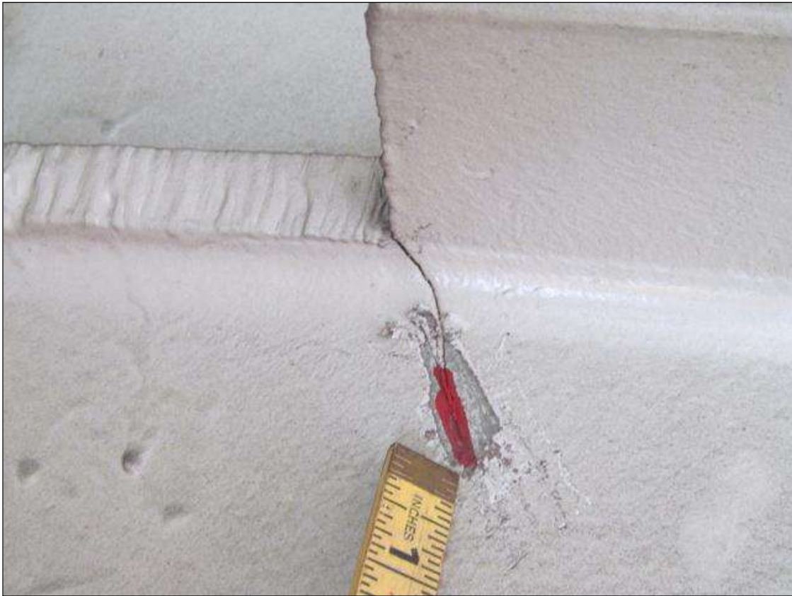
CRACK ( 3" ) IN TOP OF DIAPHRAGM. BEAM 4, SPAN 3
