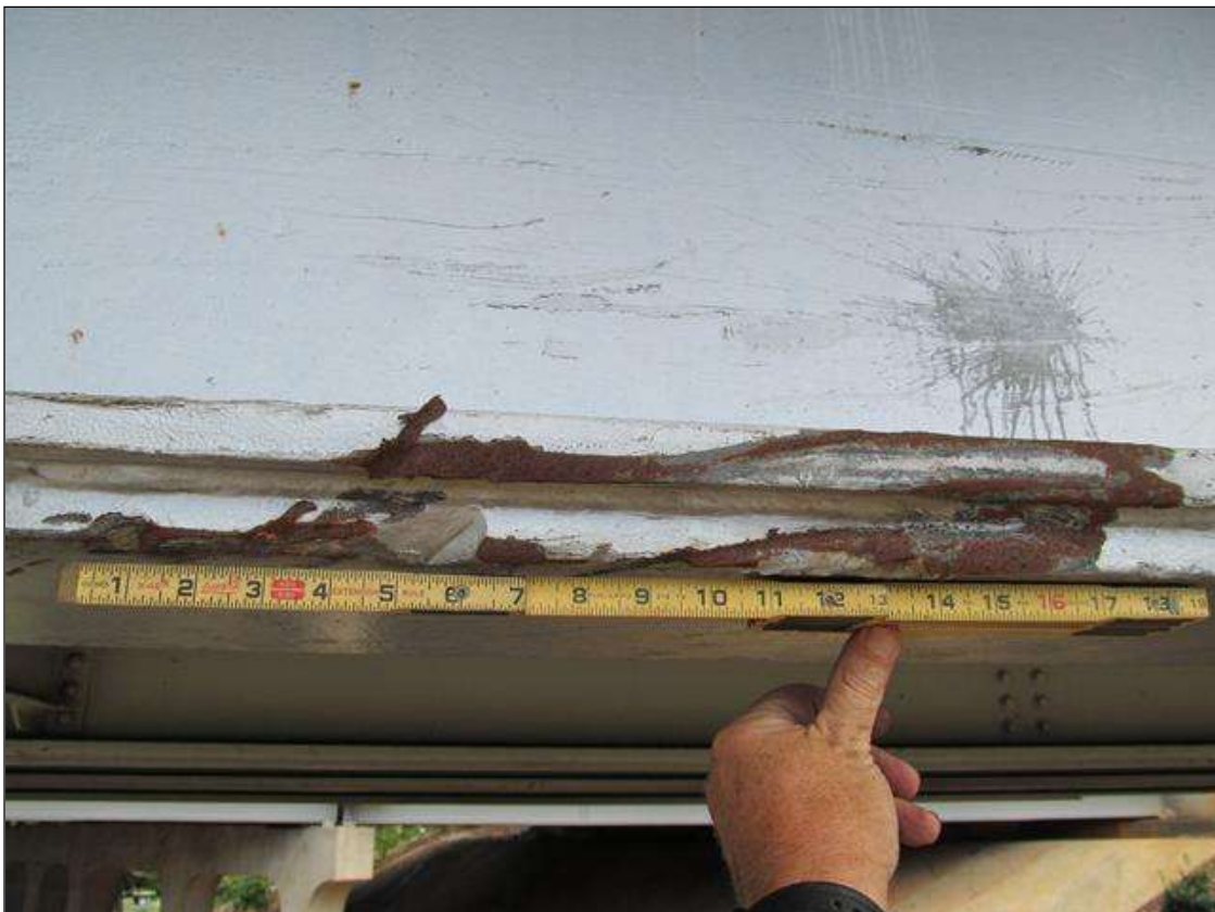
INDENTIONS IN FLANGE AND COVER PLATE @ 16'-2" FROM THE FACE OF BENT 2. BEAM 4, SPAN 3
