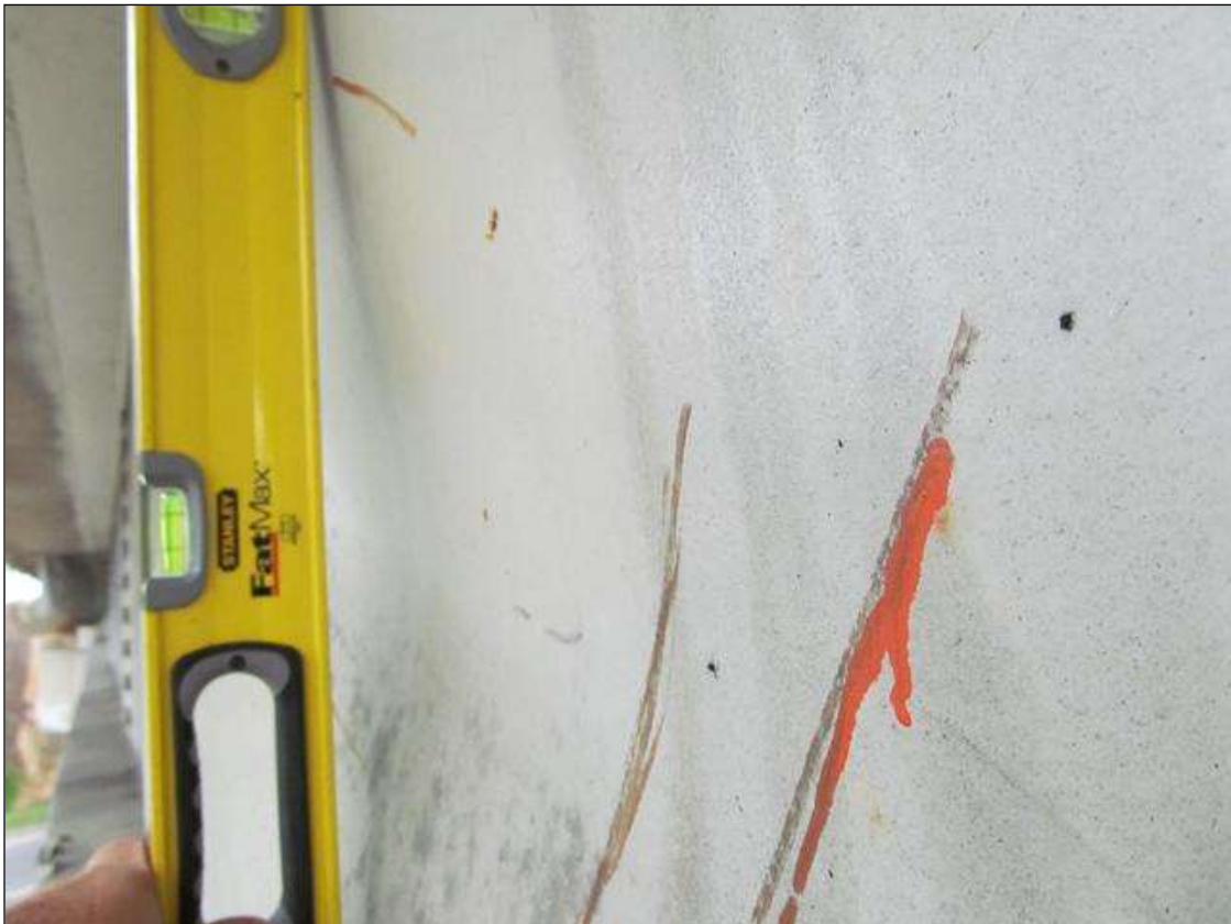
WEB OF BEAM 4 IS BENT ( 1 \frac{1}{2} " ) INWARD @ 30'-4" FROM THE FACE OF BENT 3. BEAM 4, SPAN 3
