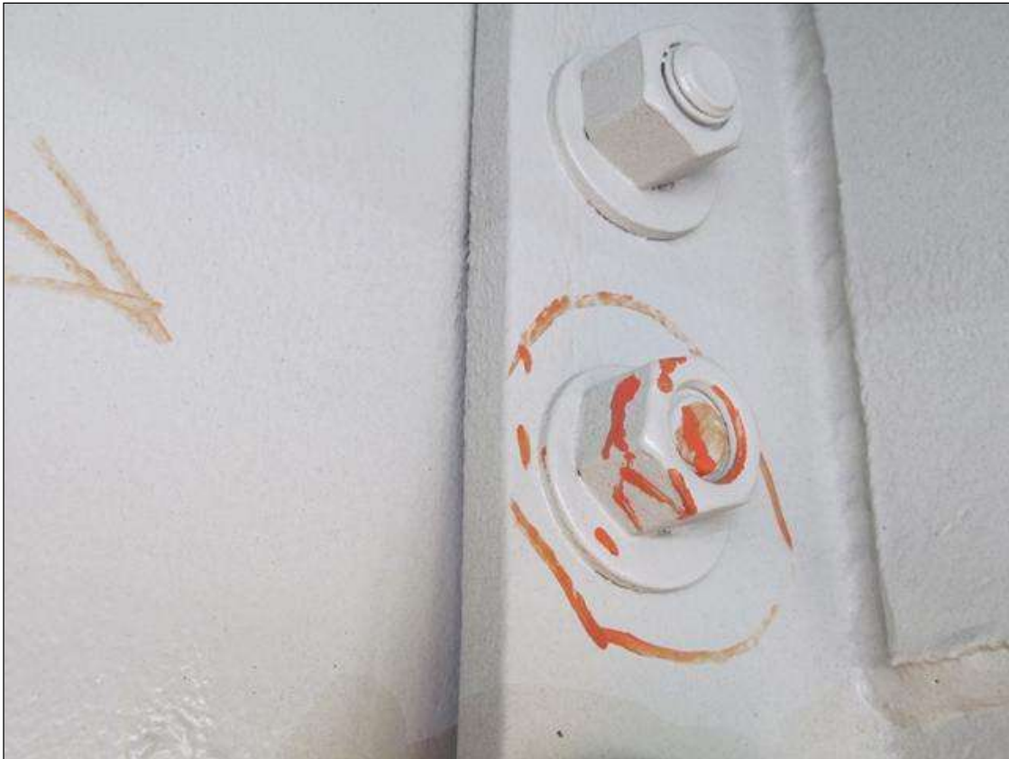
DIAPHRAGM BOLT DOES NOT HAVE A FULL THREAD @ 39'-11" FROM THE FACE OF BENT 1. GIRDER 10
