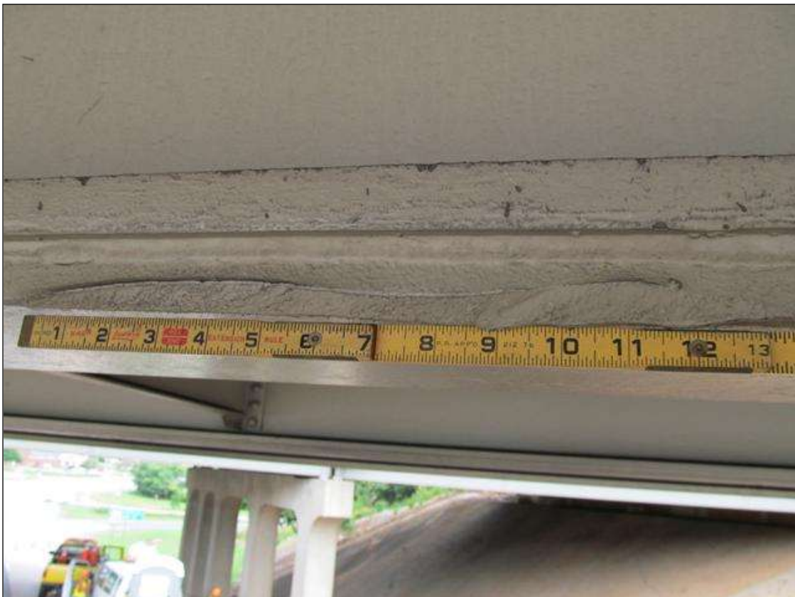
POINT OF IMPACT ON BEAM 3 IS 33'-3" FROM THE FACE OF BENT 3. BEAM 3, SPAN 3
