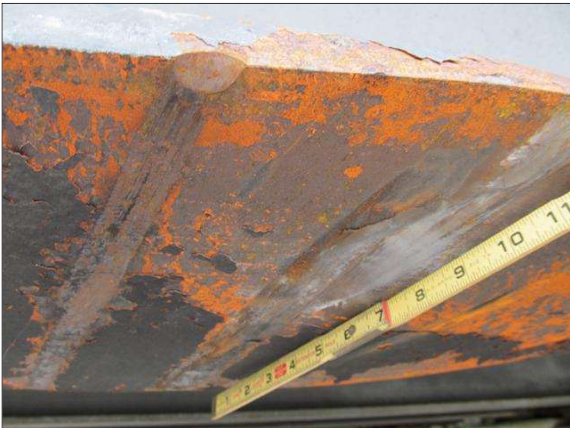
GOUGE IN BEAM 6 AT 14'-1"
