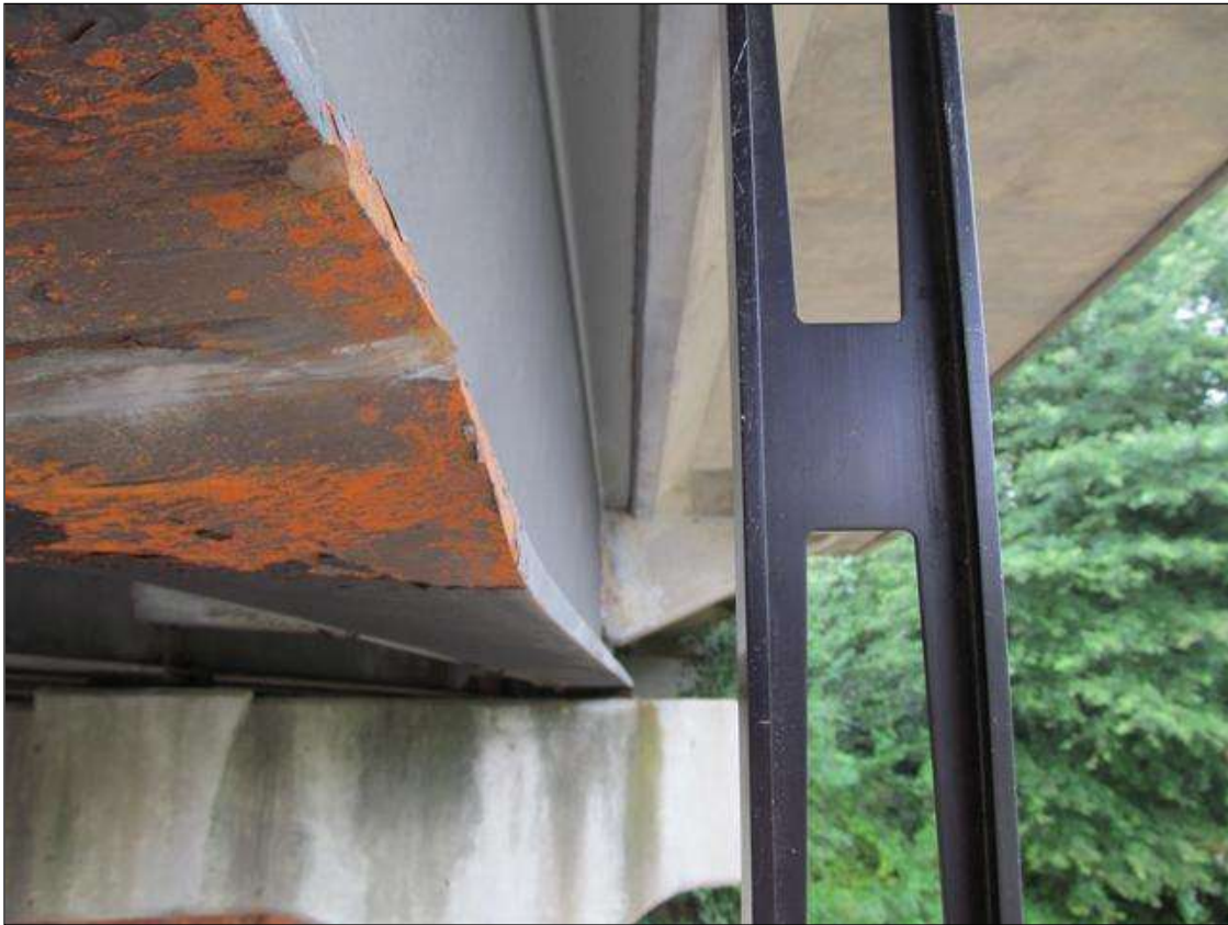
BEAM 6 OUT OF PLUMB
