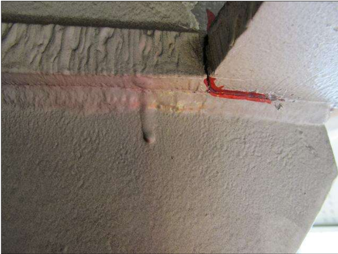
CRACK IN BOTTOM WELD OF DIAPHRAGM @ 37'-4" FROM THE FACE OF BENT 3. BEAM 4, SPAN 3
