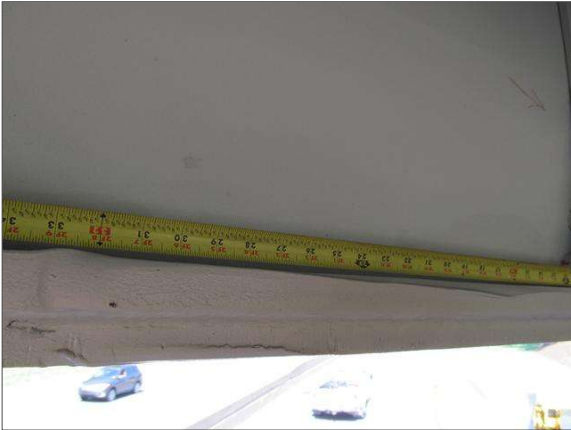
INDENTION ( 2'-10" X 1/4" ) IN FLANGE OF GIRDER 10 @ 43'-1" FROM THE FACE OF BENT 1 AND COVER PLATE ( 7" X 1/16" )
