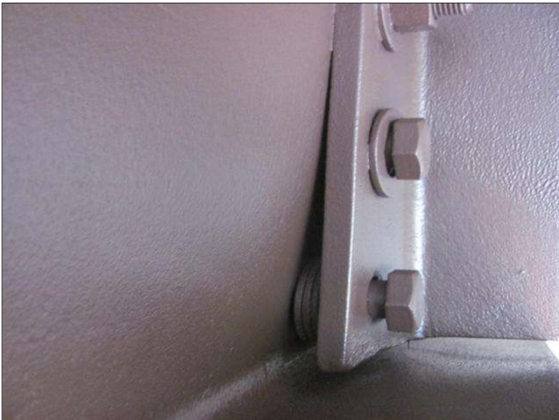
FOUR DIAPHRAGM BOLTS ARE NOT TIGHT @ 19'-4" FROM THE FACE OF BENT 1. GIRDER 10
