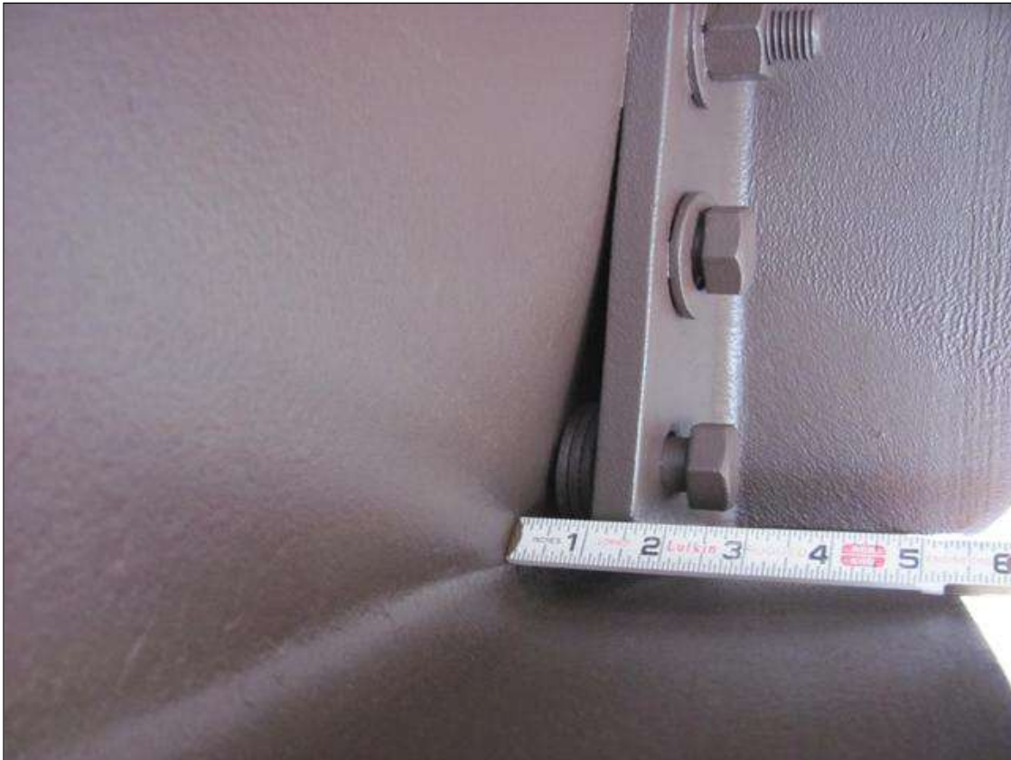
BOTTOM OF WEB IS BENT TO THE SOUTH 7/8" AT DIAPHRAGM @ 19'-4" FROM THE FACE OF BENT 1. GIRDER 10
