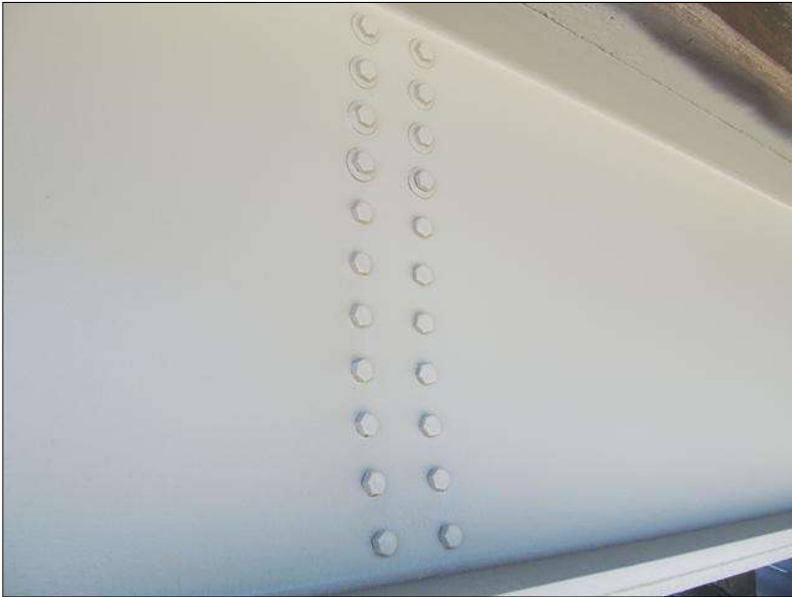
14 DIAPHRAGM BOLTS WITHOUT WASHERS AND 8 WITH WASHERS @ 39'-11" FROM THE FACE OF BENT 1. GIRDER 10
