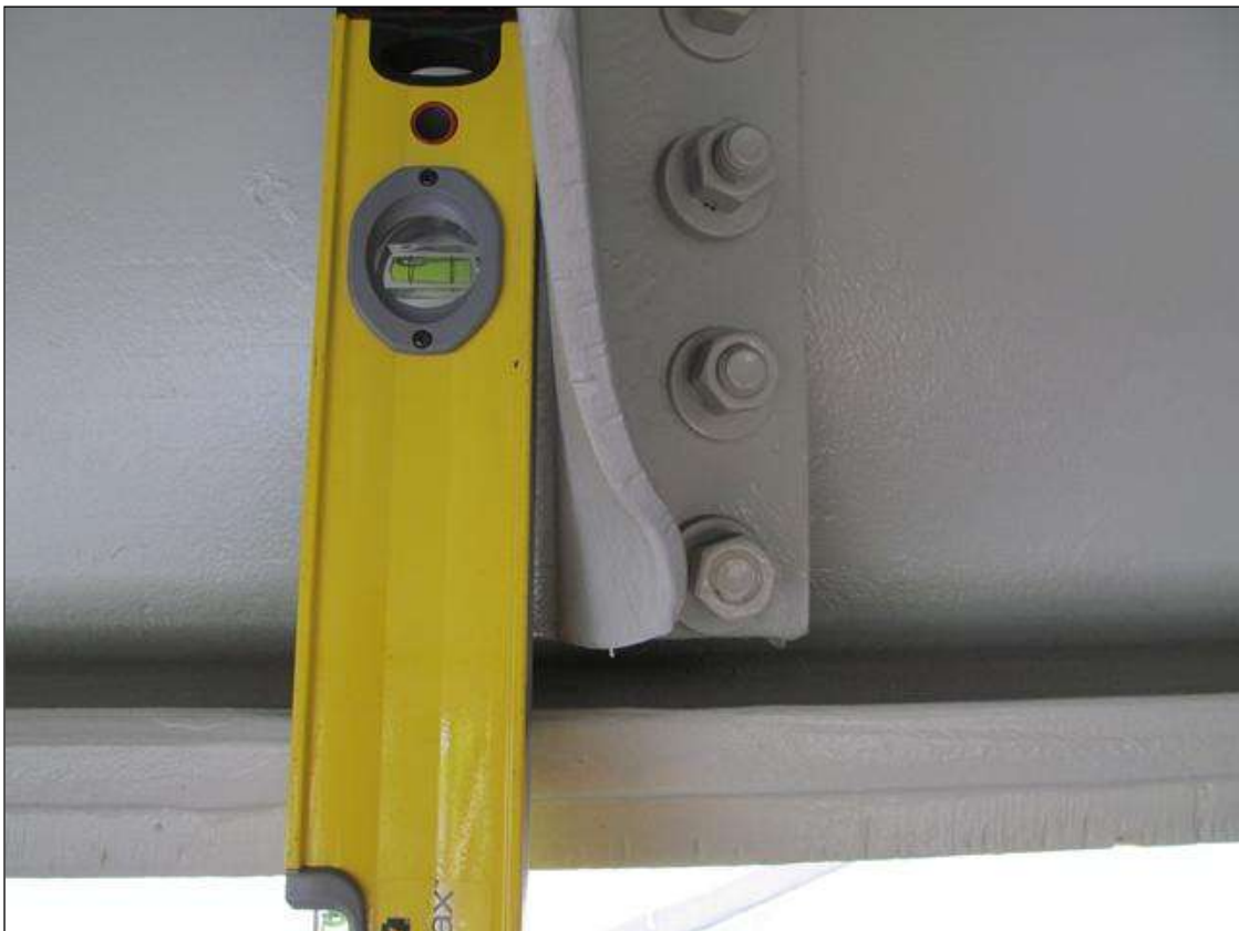
DIAPHRAGM BRACE IS BENT ( 1 1/4" ) TO THE WEST @ 39'-11" FROM THE FACE OF BENT 1. GIRDER 10
