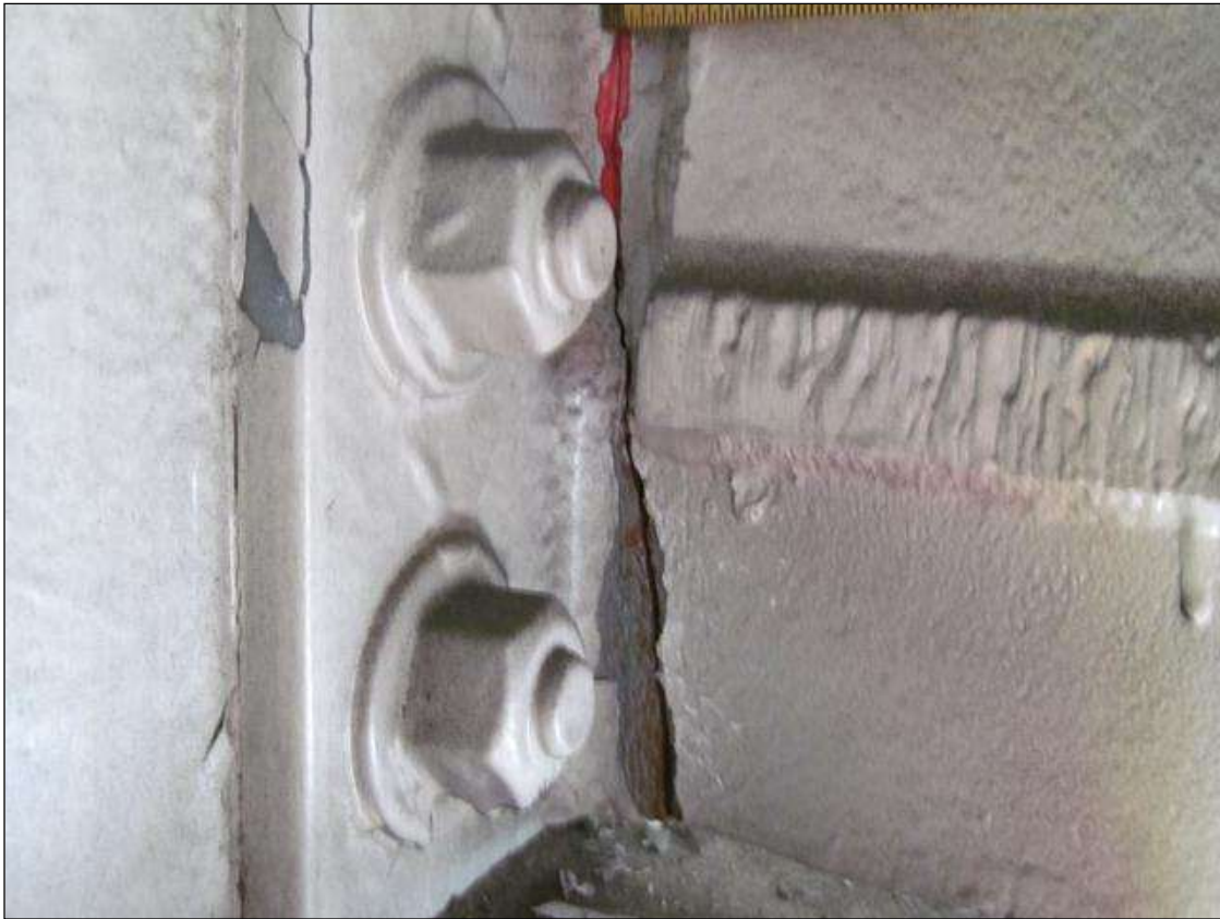
CRACK ( 6 1/2" ) IN BOTTOM OF DIAPHRAGM BRACKET. BEAM 4, SPAN 3
