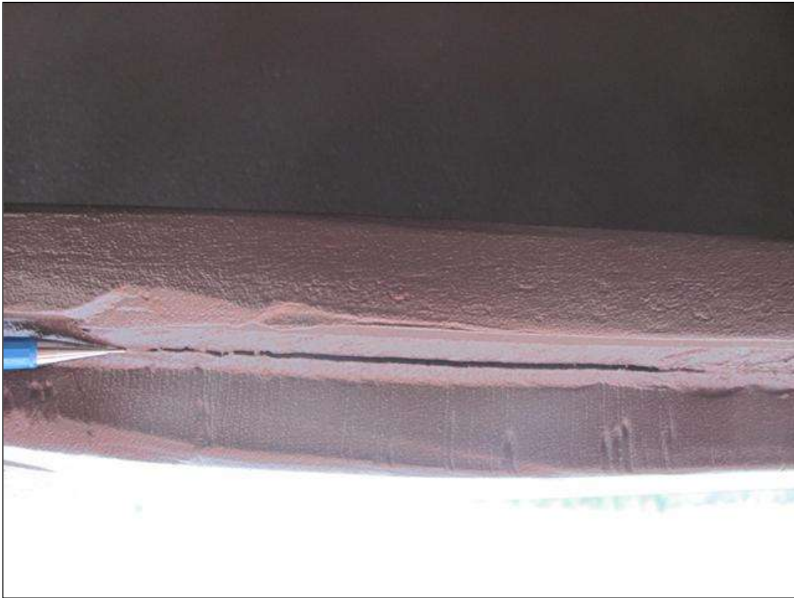
CRACK 8" LONG IN WELD OF COVER PLATE TO FLANGE @ 21'-2" IN GIRDER 10
