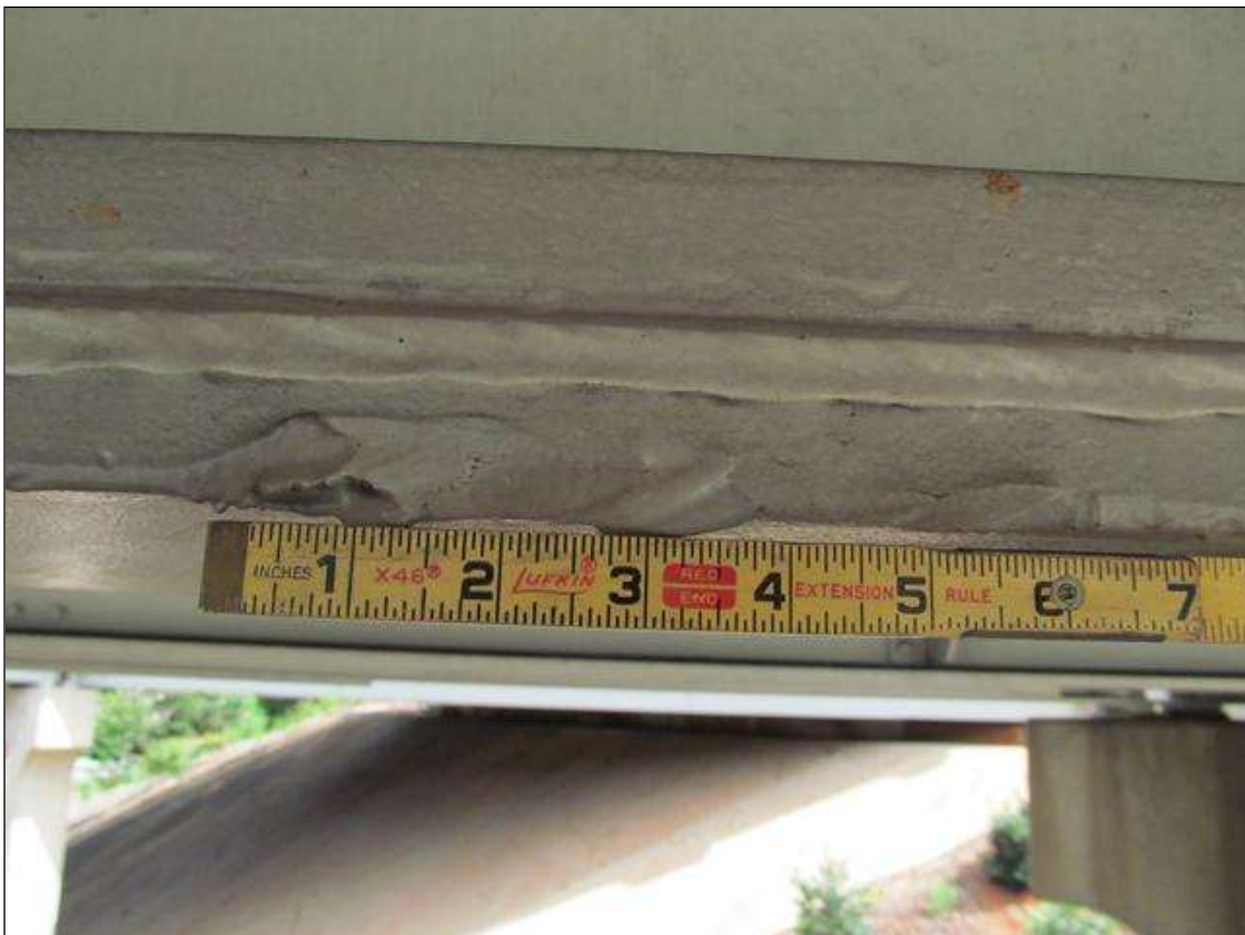
INDENTATION ( 6" X 1/4" ) IN COVER PLATE @ 23'-2" FROM THE FACE OF BENT 3. BEAM 3, SPAN 3
