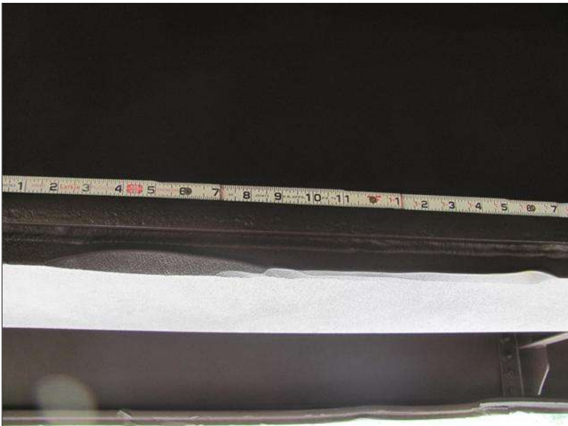
POINT OF IMPACT ON GIRDER 9 WAS 18'-0" FROM THE FACE OF BENT 1. INDENTIONS IN COVER PLATE
