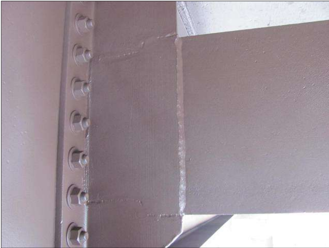
REPAIRS MADE TO DIAPHRAGM @ 16'-6" ON SOUTH SIDE OF GIRDER 9
