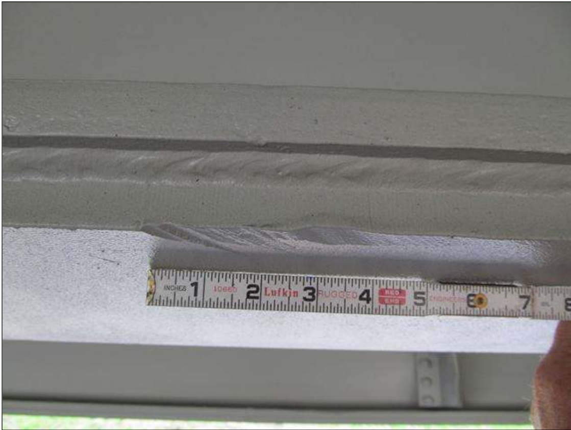
POINT OF IMPACT, IN MIDDLE LANE, ON GIRDER 9 IS 36'-6" FROM THE FACE OF BENT 1. INDENTATION IN COVER PLATE IS 5" X 1/16".
