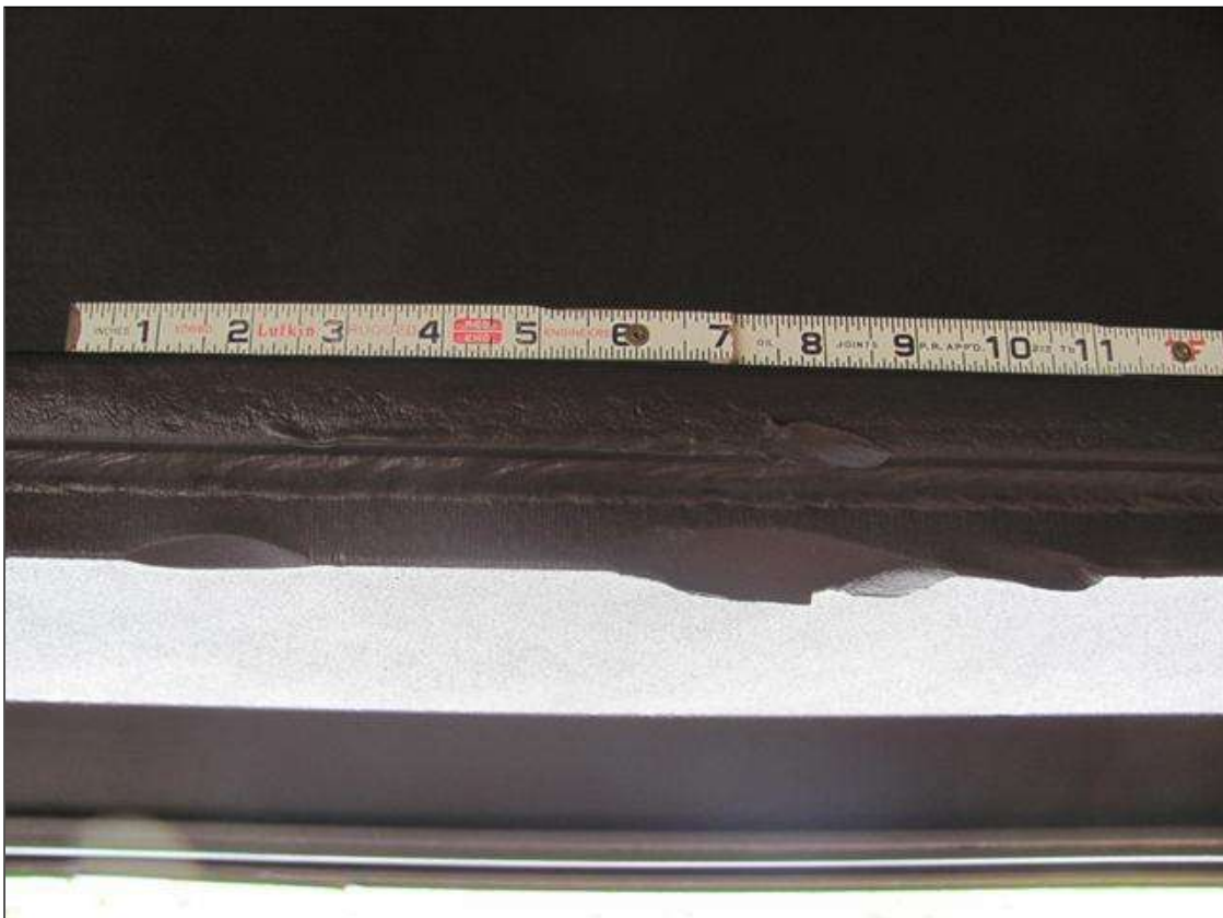
IMPACT ON GIRDER # 8 WAS 21'-6" FROM THE FACE OF BENT 1.
