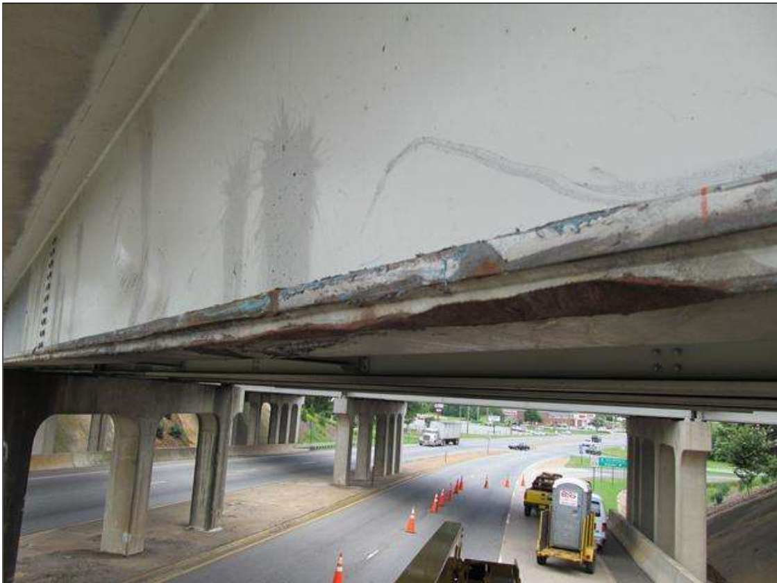
LOOKING AT BEAM 4 FROM BENT 3. BEAM 4 FLANGE AND COVER IS DAMAGED
