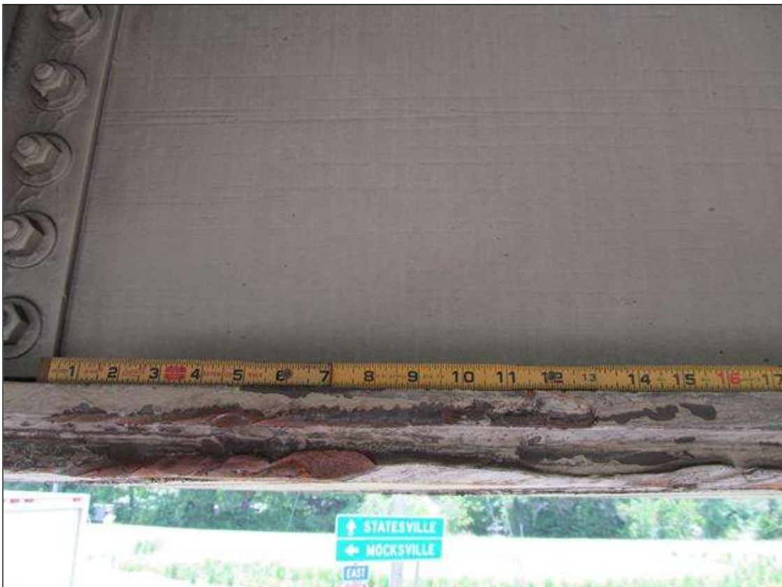
POINT OF IMPACT ON BEAM 4 @ 19'-1" FROM THE FACE OF BENT 2. BEAM 4, SPAN 2
