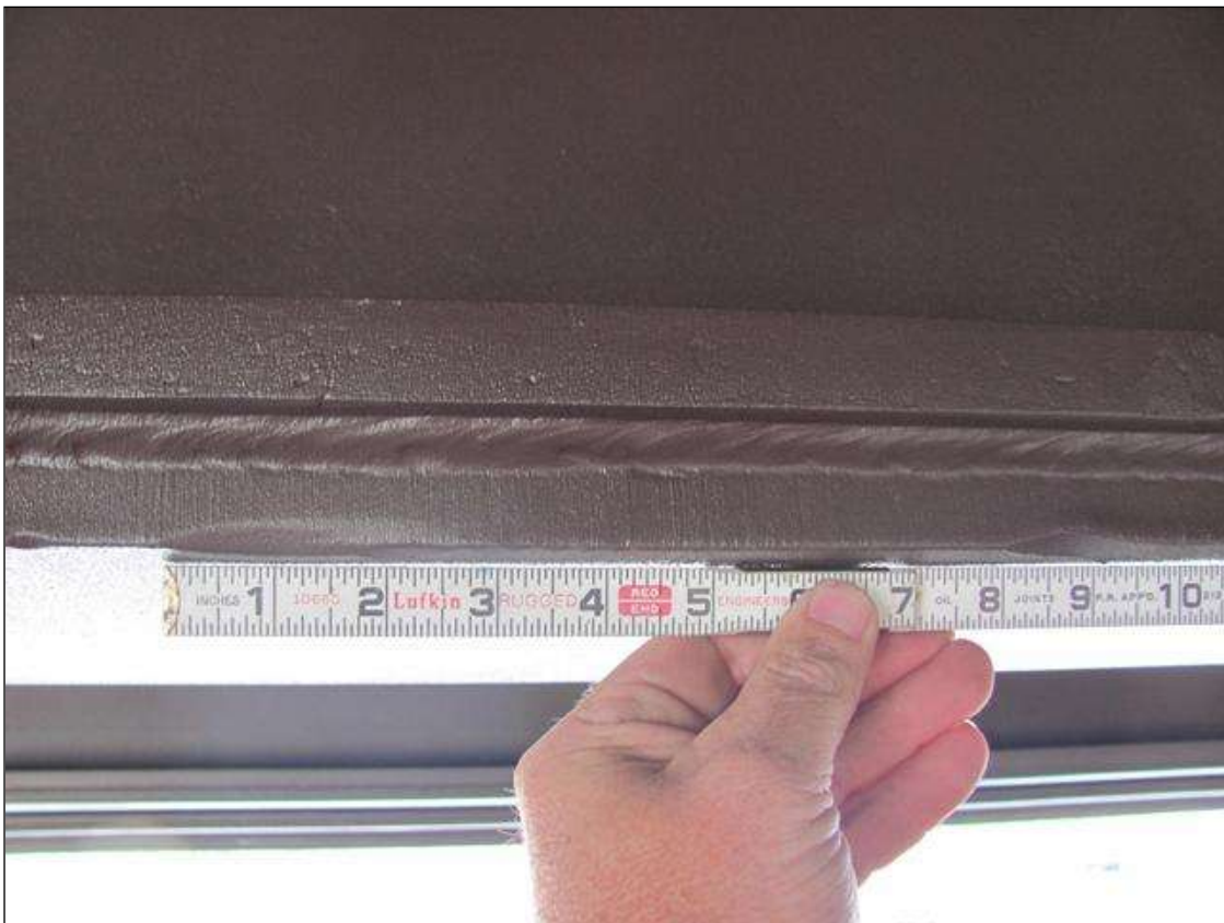
IMPACT ON GIRDER # 6 WAS 23'-6" FROM THE FACE OF BENT 1. INDENTIONS 2 1/2" X 1/16" & 4" X 1/16"
