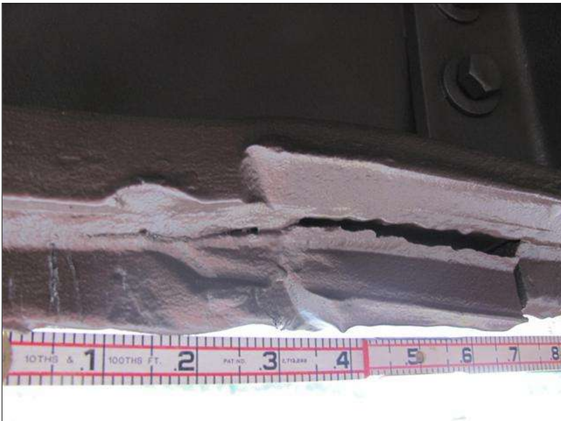
CRACK IN WELD IN COVER PLATE TO FLANGE IS 1 FOOT LONG @ 19'-11" FROM THE FACE OF BENT 1 GIRDER 10
