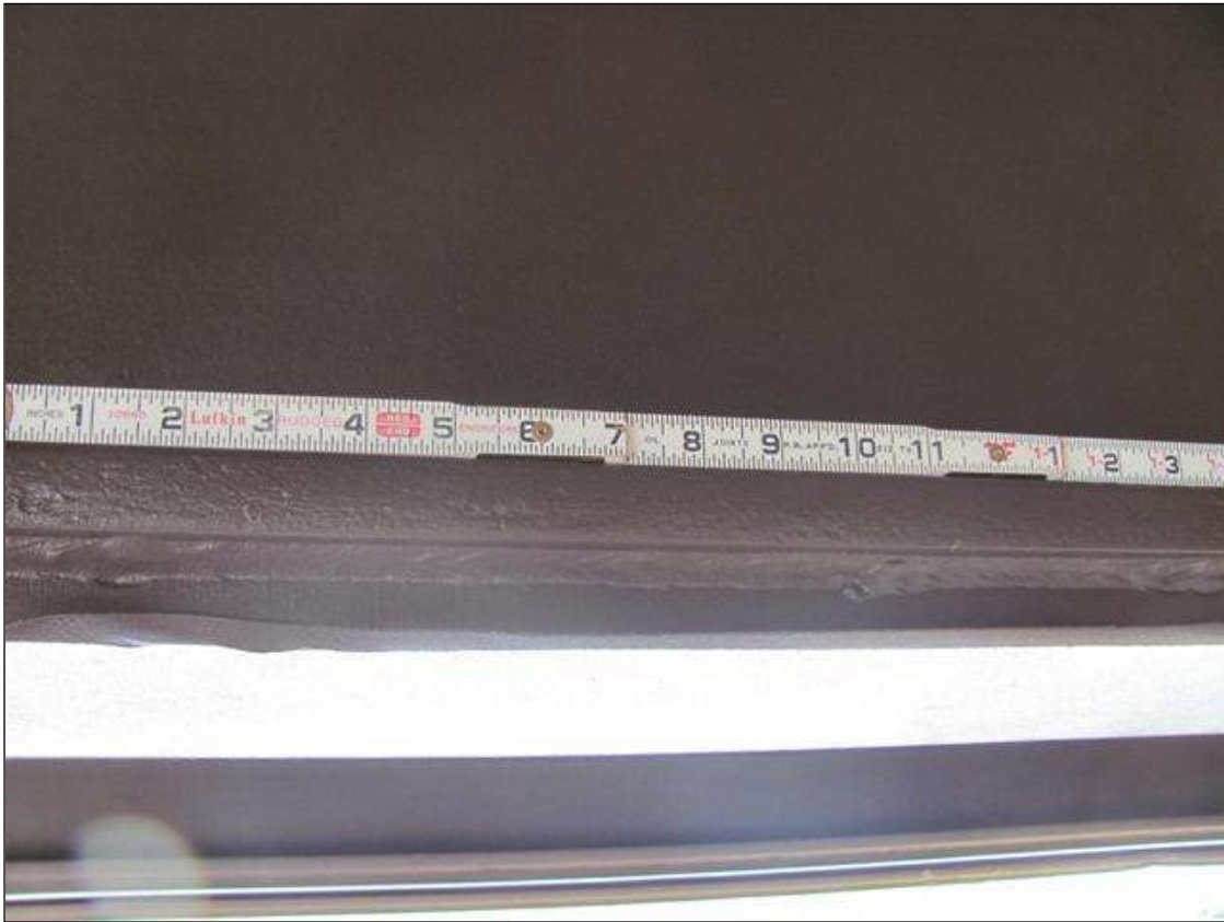
INDENTION ( 1'-7" X 1/16" ) IN COVER PLATE @ 19'-4" FROM THE FACE OF BENT 1. GIRDER 8
