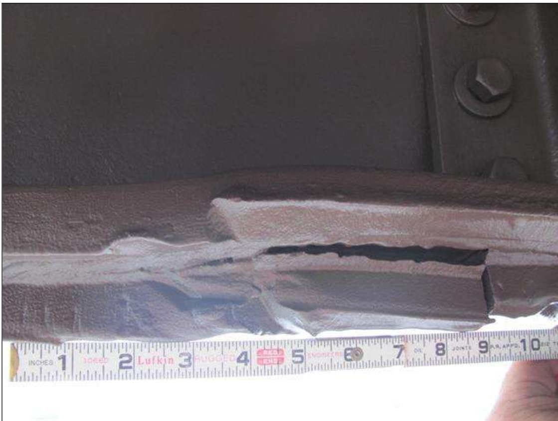
IMPACT ON GIRDER 10 WAS 19'-11" FROM THE FACE OF BENT 1.
