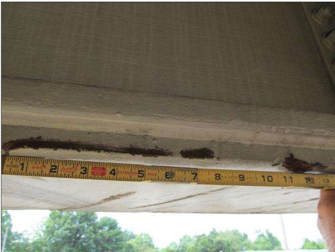
INDENTIONS IN COVER PLATE ON NORTH SIDE OF BEAM 4 @ 36'-3" FROM THE FACE OF BENT 3. BEAM 4, SPAN 3
