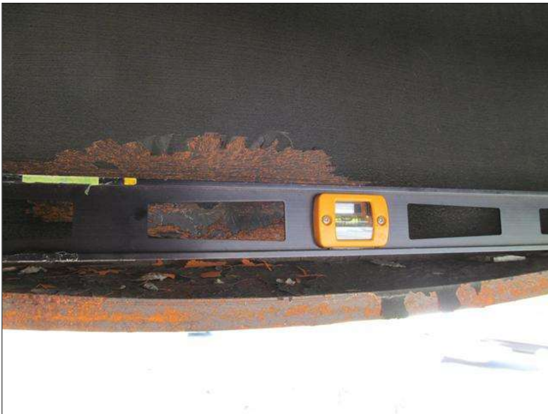
FLANGE ON BEAM 6 BENT DOWN
