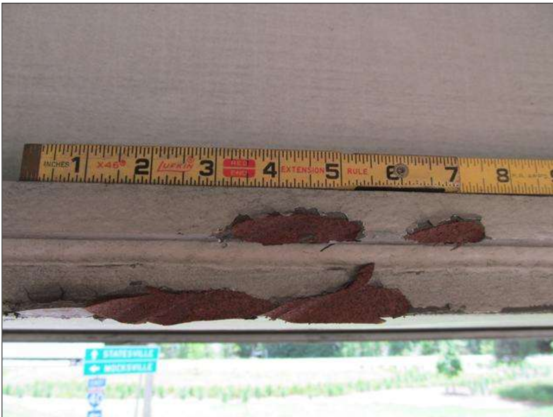
POINT OF IMPACT ON BEAM 3 @ 20'-2" FROM THE FACE OF BENT 2. BEAM 3, SPAN 2
