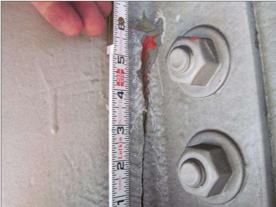
CRACK ( 6" ) IN BOTTOM OF DIAPHRAGM @ 37'-4" FROM THE FACE OF BENT 3. BEAM 4, SPAN 3
