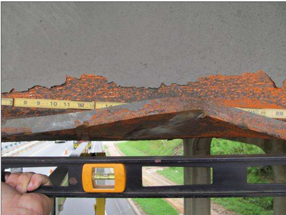
DAMAGE TO BEAM 6 AT 14'-1"
