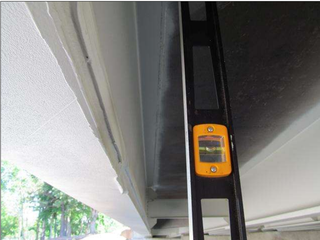
GIRDER 10 IS OUT OF PLUMB ( 4 1/4" ) @ 37'-5" FROM THE FACE OF BENT 1
