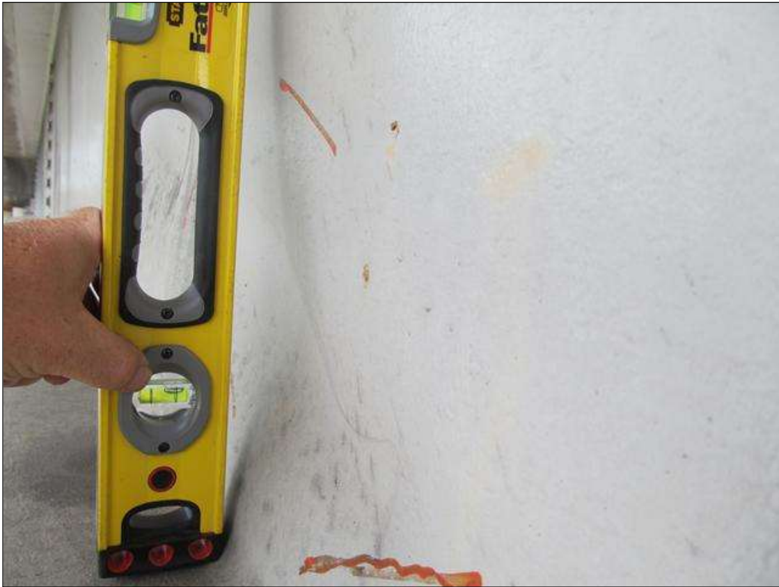
WEB OF BEAM 4 IS BENT ( 1 1/4" ) INWARD @ 28'-6" FROM THE FACE OF BENT 3. BEAM 4, SPAN 3
