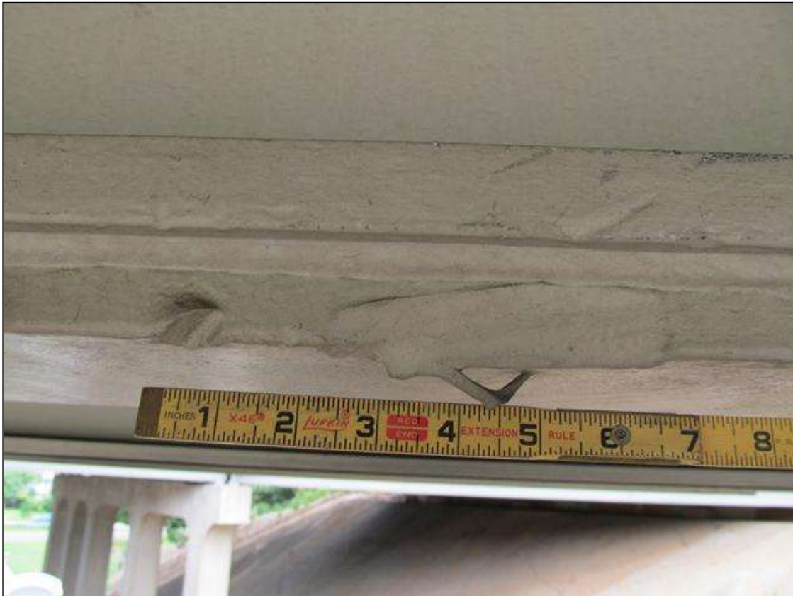
INDENTATION ( 1/2" X 1/4" ) IN COVER PLATE @ 35'-1" FROM THE FACE OF BENT 3. BEAM 3, SPAN 3
