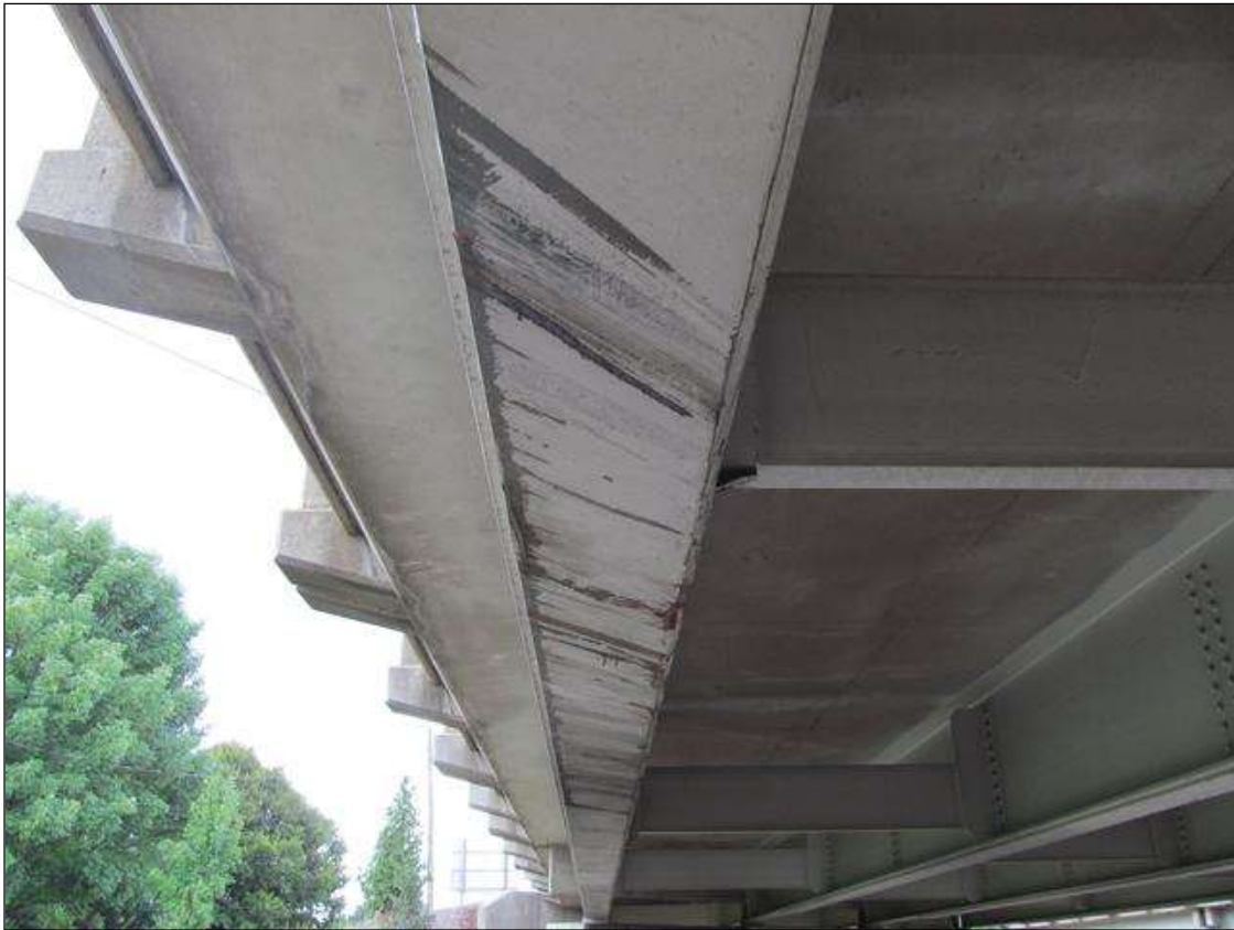
MARKS AND SCRAPES ON COVER PLATE TO BEAM 4, SPAN 2
