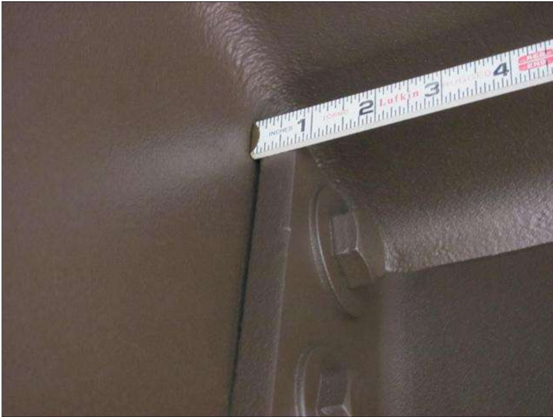
TOP OF DIAPHRAGM @ 13'-11" HAS PULLED AWAY FROM FLANGE 1/8". GIRDER 9
