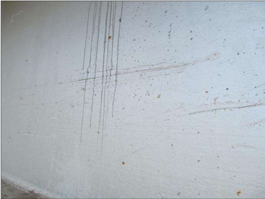
MARKS ON WEB HAVE BEEN PAINTED OVER. BEAM 4, SPAN 3
