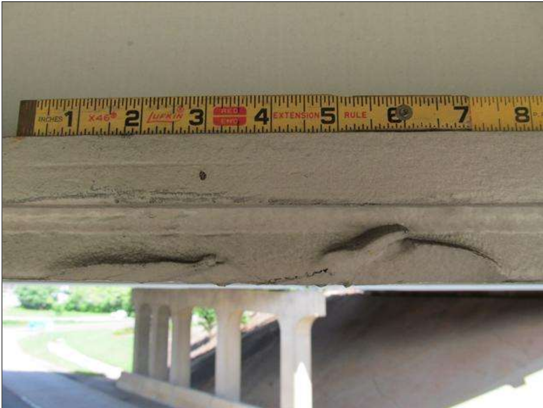
INDENTION ( 8" X 1/4" ) IN COVER PLATE @ 15'-5" FROM THE FACE OF BENT 2. BEAM 3, SPAN 3
